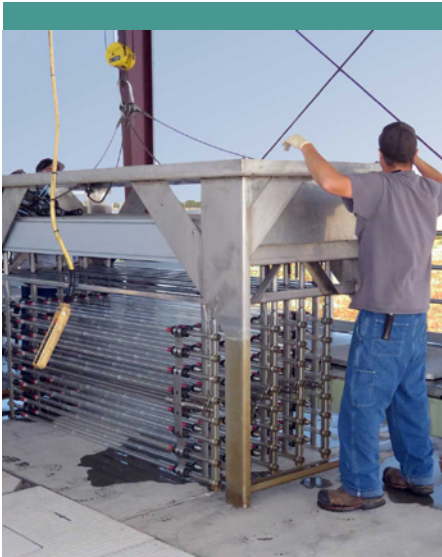
UV Lights at the Water Recycling Facility
