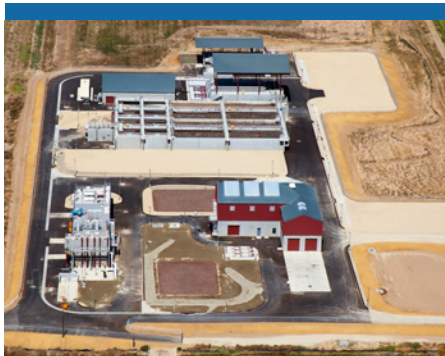
Water Recycling Facility
