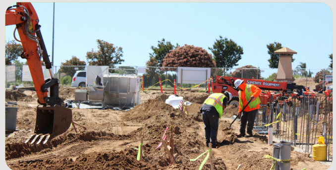
ISD staff inspected the installation of sewer pipes to accommodate a new business, supporting economic development and the Community's continued growth.
