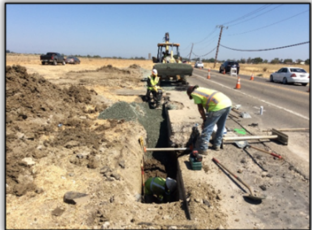
Sewer construction project.
