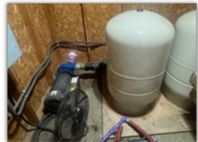
Installation of a recycled water pump station.
