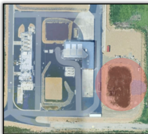
Stormwater retention pond (circled in red).
