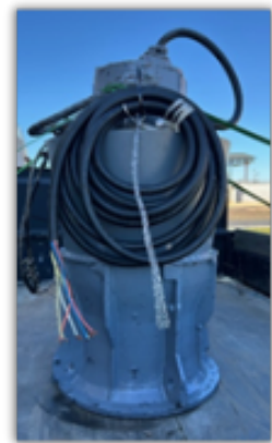
Sludge Pump after rehab.
