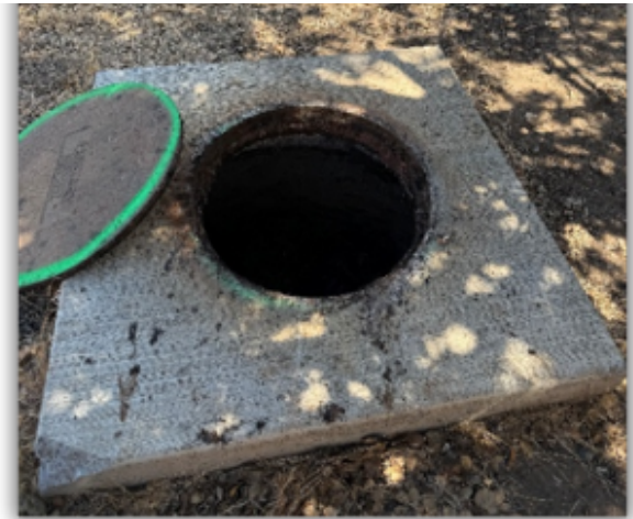
Manhole cover and frame.
