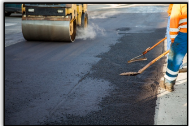
Asphalt being applied after gravity pipeline replacement.
