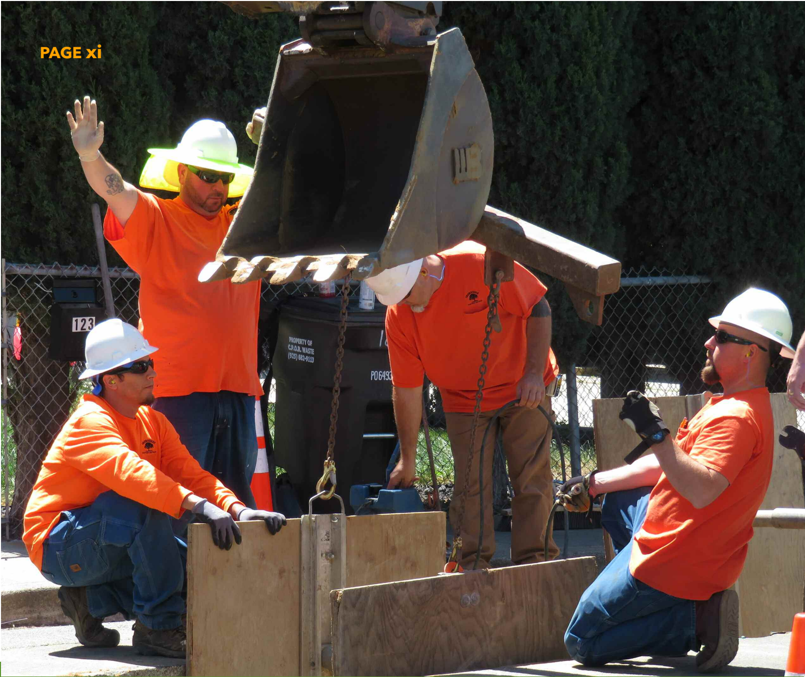
Ironhouse Collections crews working setting up safety precautions before working underground.
