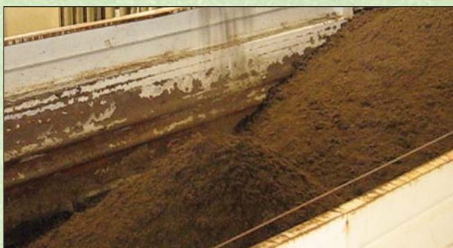
Biosolids are collected for distribution at ISD's Water Recycling Facility.
