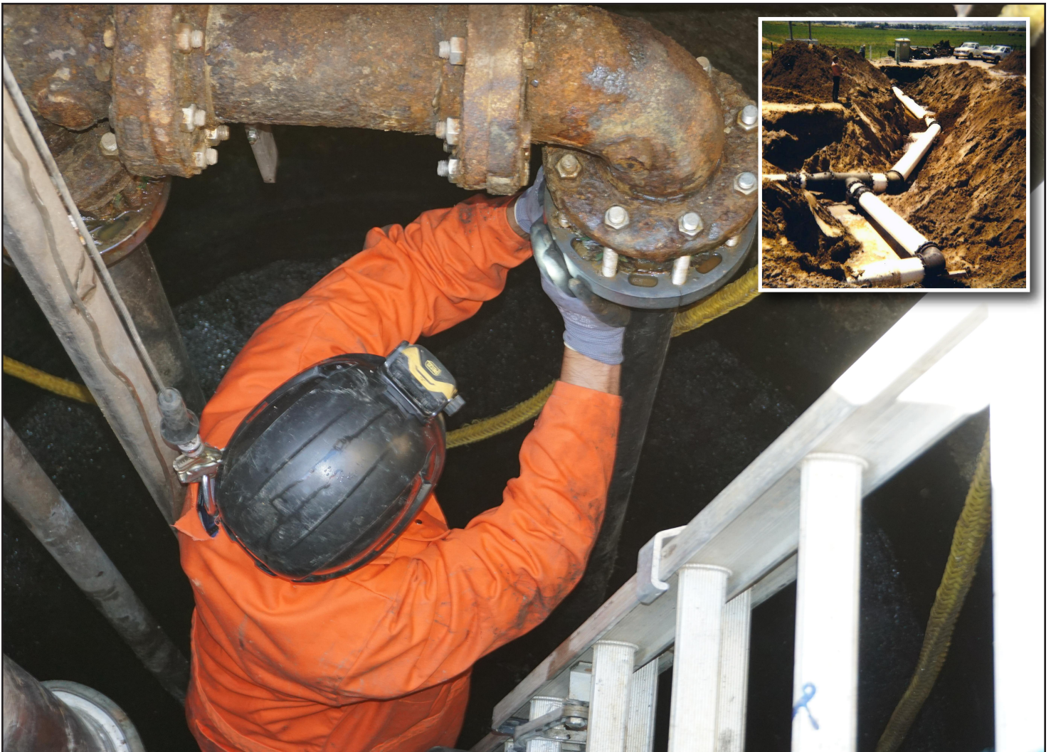
Ironhouse Collections crews working on a confined space project on Bridgehead Road in Oakley. (Insert photo) Oakley Sanitary District collection crews working a pipe project in Oakley during the 1980s.
