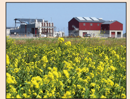
Water Recycling Facility to receive major upgrades.
