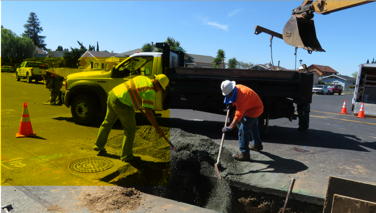
Ironhouse Collections crew cleaning up confined entry space after replacing a clay sewer pipe installed in the 1940s.
